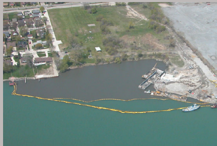
Through the Great Lakes Legacy Act, more than 470,000 pounds of contaminated sediment were removed.
