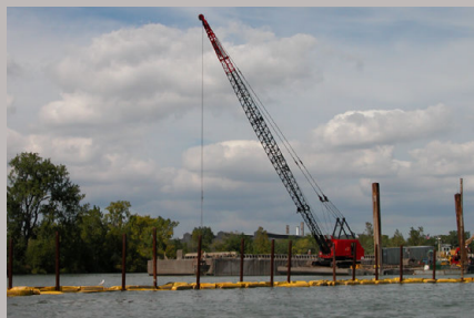
Heavy machinery was required to remove the oil and grease from the bed of the inlet.
